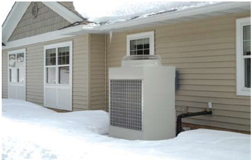
The CITY MULTI® VRFZ System installed at the Brentwood assisted living facility provides individual and simultaneous cooling and heating to 29 units, the kitchen and a chapel.
